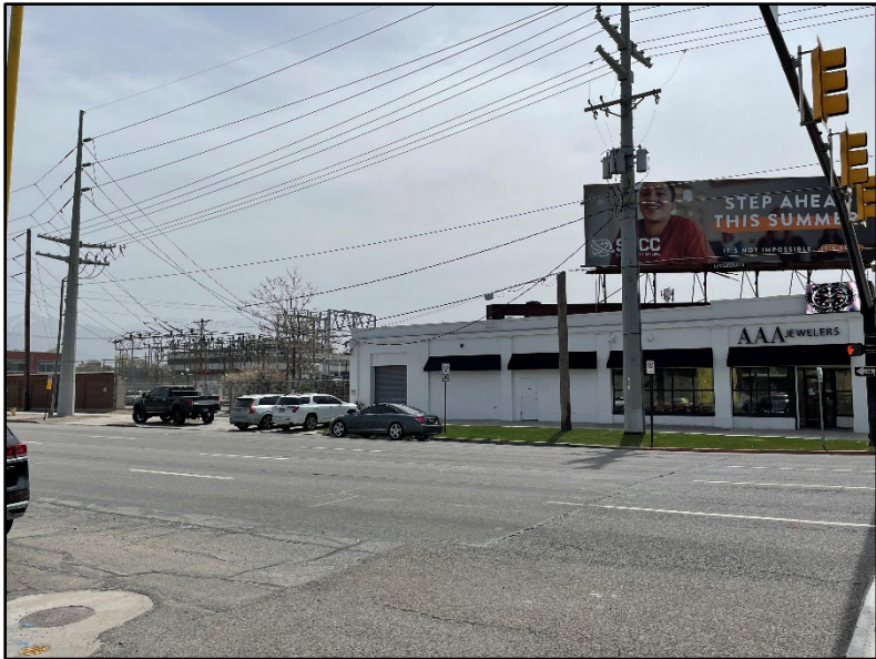
Rocky Mountain Power substation and Adjacent Business
