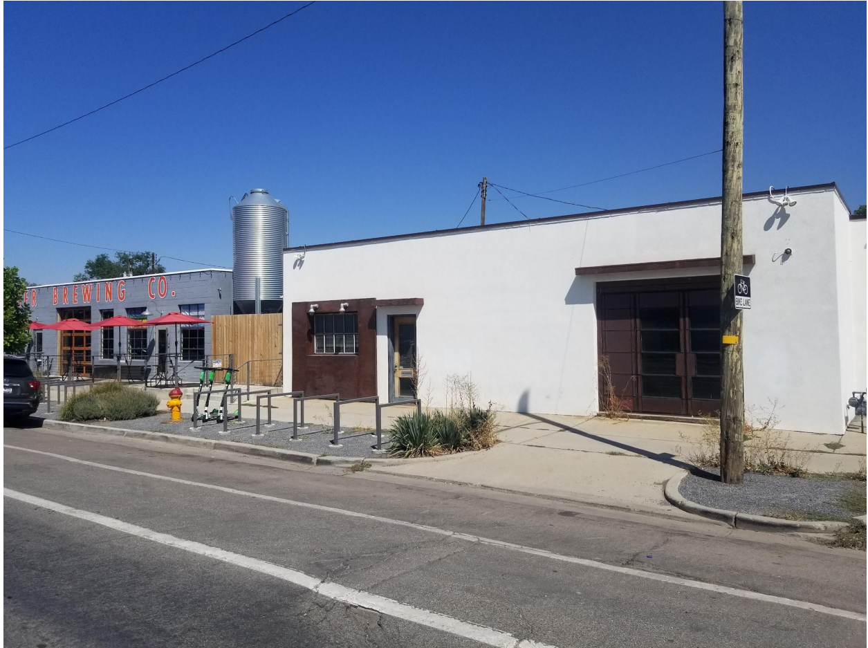
Photo 1: Existing Fisher Brewing Co. Building with Silo and side patio gate and south facade of expansion building at 778 S. 300 W. (white). This curb cut would be removed and replaced with a tree and the building itself would be painted grey to match the existing brewery with signage/logos/murals/ etc. possible in the large blank areas of the facade.
