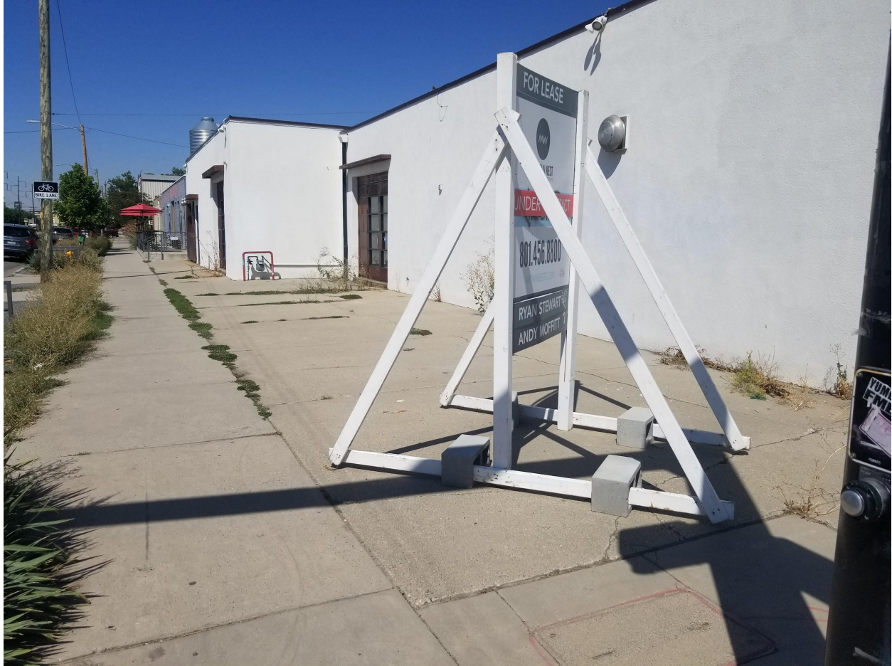
Photo 3: Existing SW Side/Front Yard area to be utilized with a patio for patrons including railings, patio shade structures, planters and additional landscaping. Building painting, signage and lighting will also be incorporated to match the existing brewery. East facing wall provides a prime mural location.
