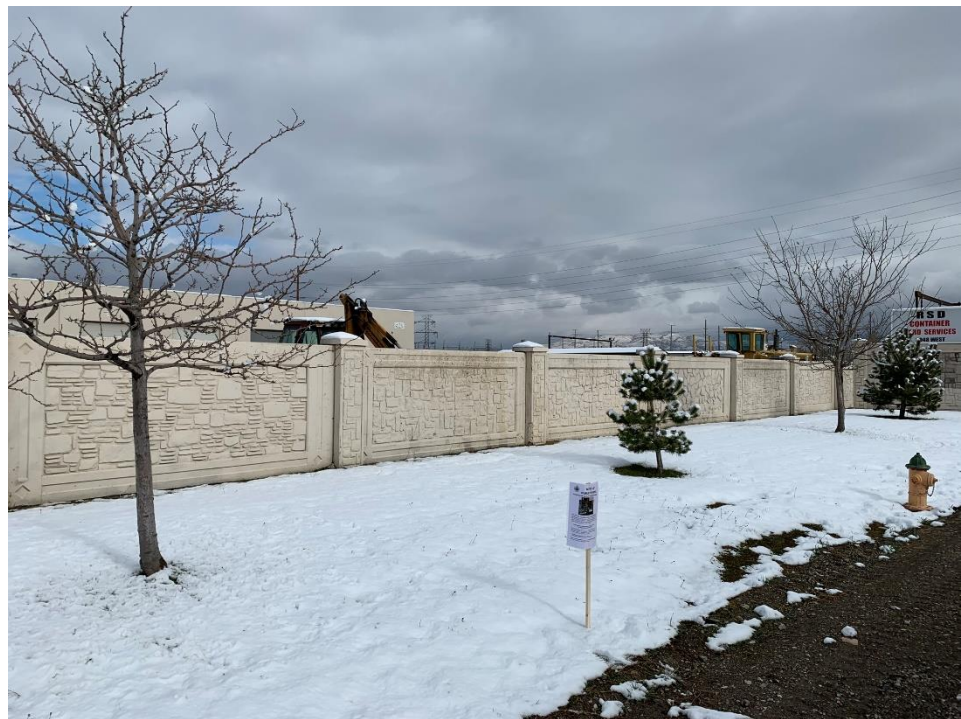
Street frontage on 700 S looking east
