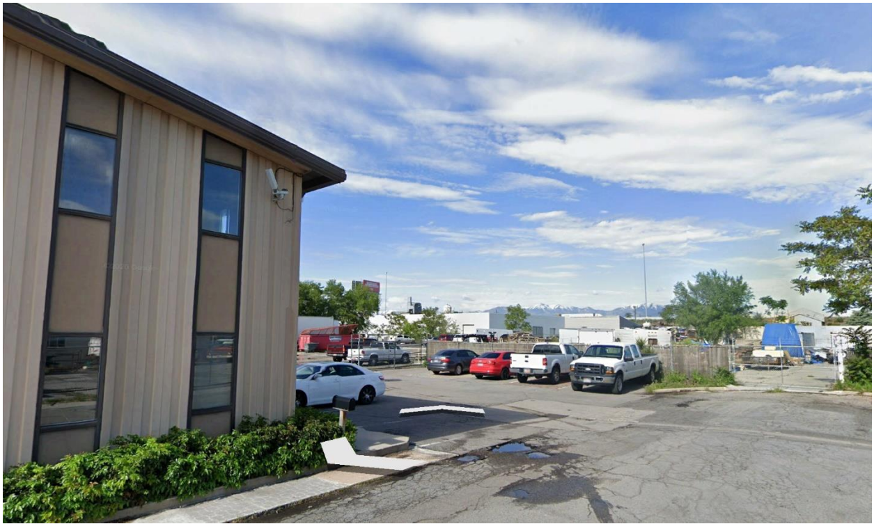
Office & Storage Area Across the Street to the South- Looking Southwest
