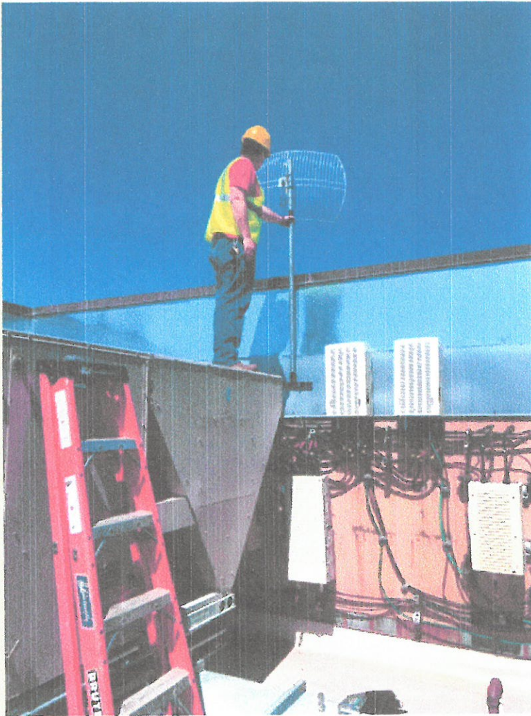
Preferred location (1) of Donor Antenna (NW view mounted to existing antenna mount.)
