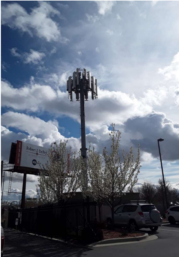
Figure 1: South Facing View of Antenna on Warm Springs Rd.
