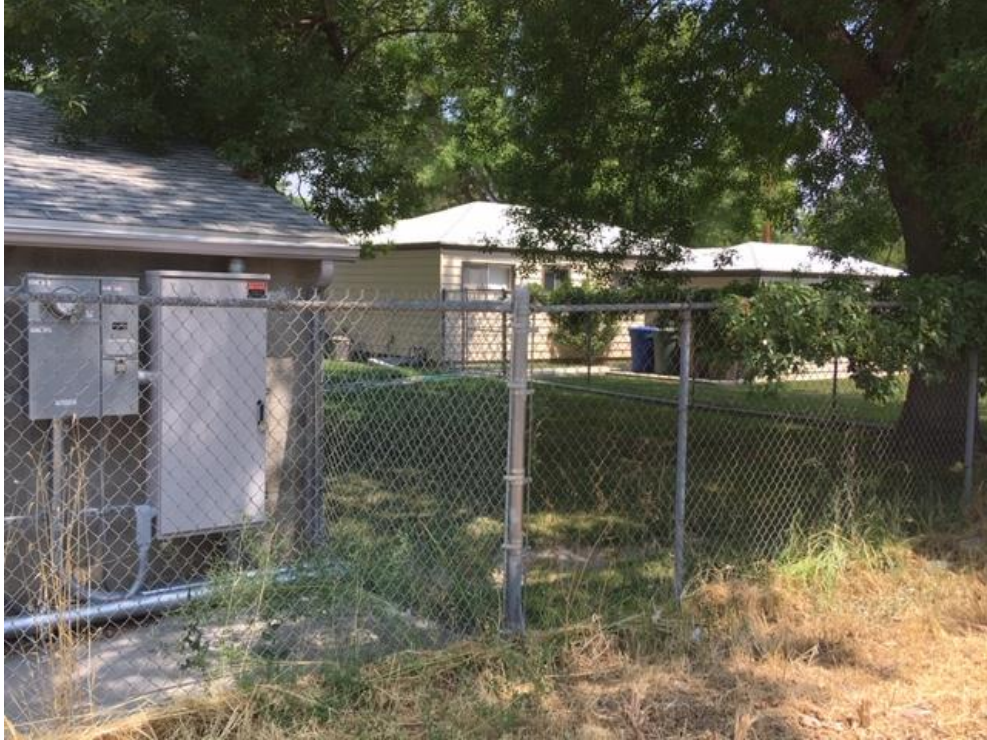
View of the shed with antenna equipment on the rear of the subject property
