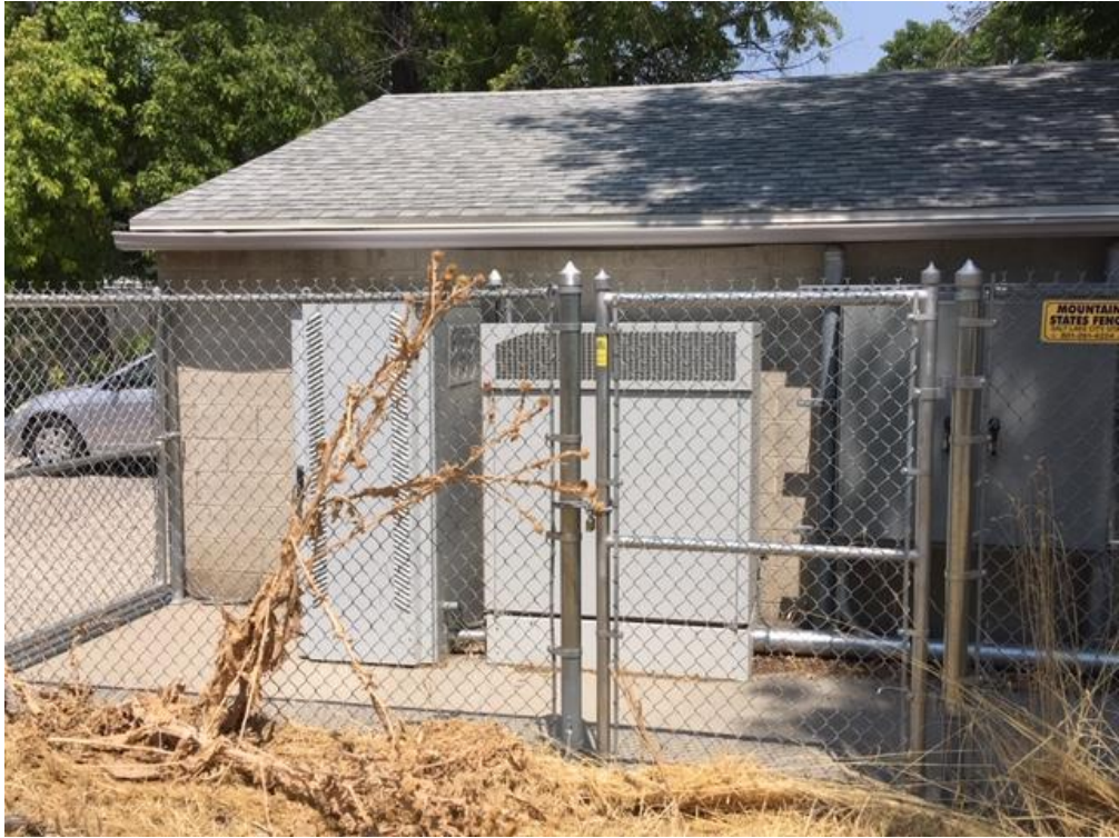
Alternate view of shed with antenna equipment
