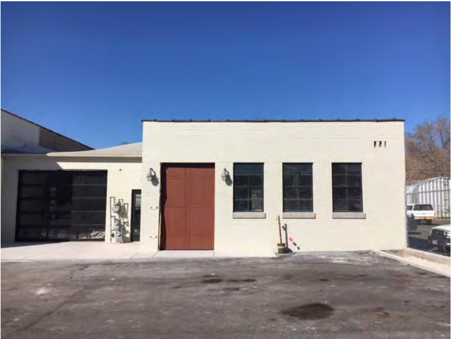
The photograph looking towards the west, shows the north portions of the building at 936 S. 300 W. This would be the main entrance into the tap room.
