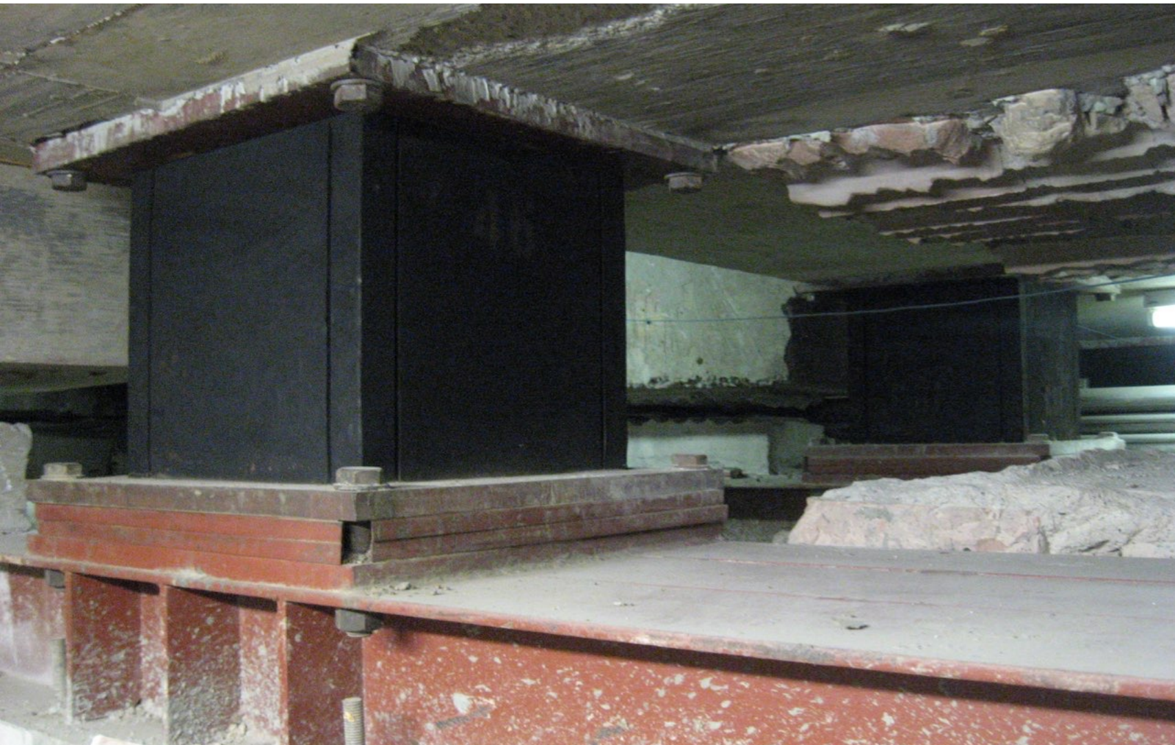
Installed base isolators
