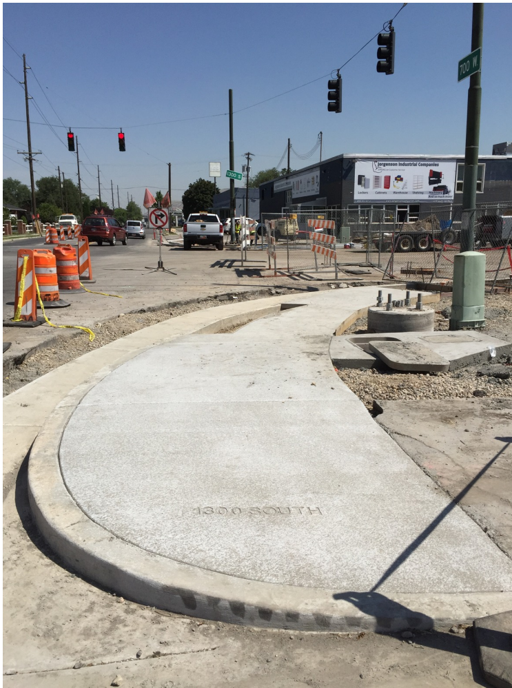
Work on the new intersection at 700 West
