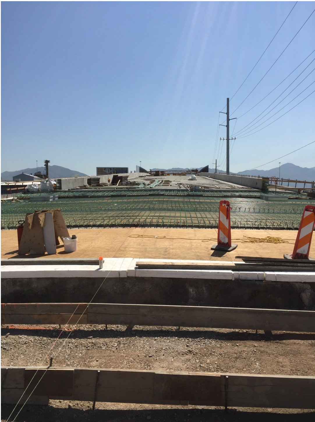
Forming the west side bridge approach
