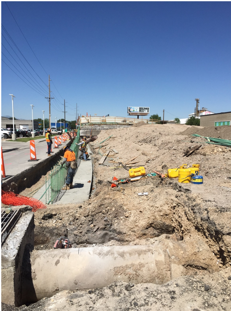
Crews forming the east side retaining walls
