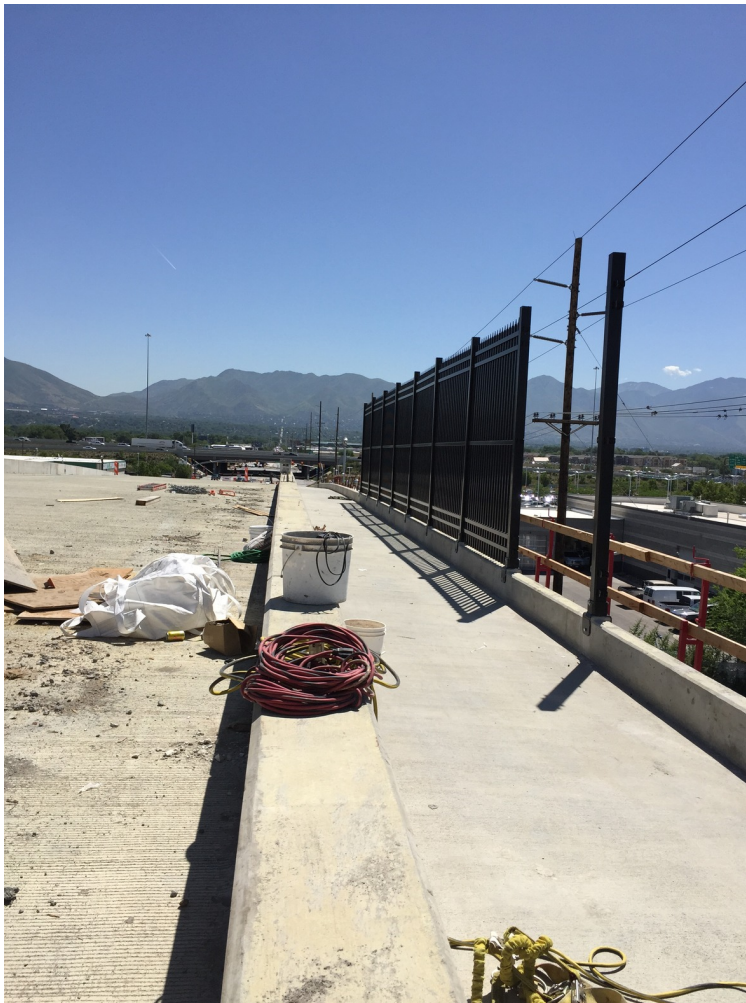
Fence installation on the bridge deck
