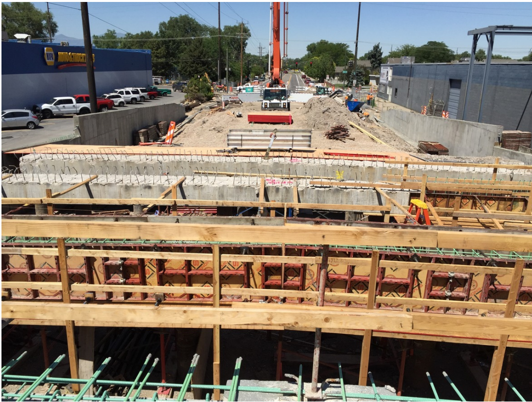
Forming the west side pile slab
