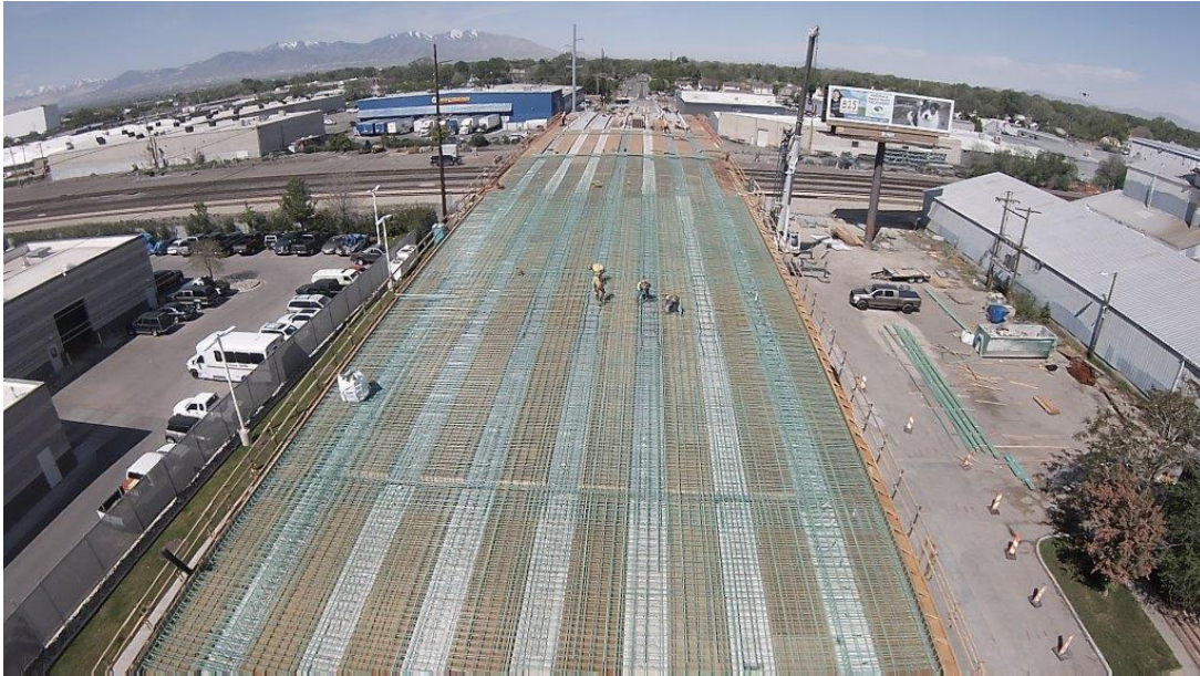
Aerial view of the project
