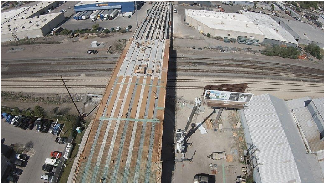
Aerial view of the project
