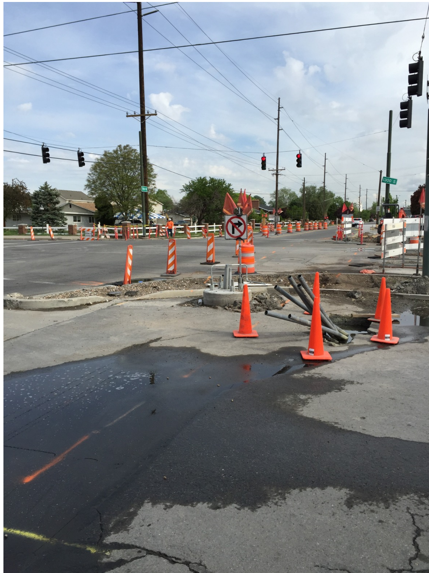
Work on the new signal at 700 West
