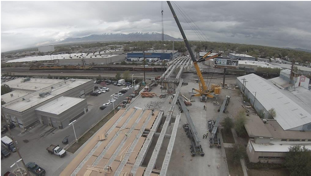
Aerial view of the project
