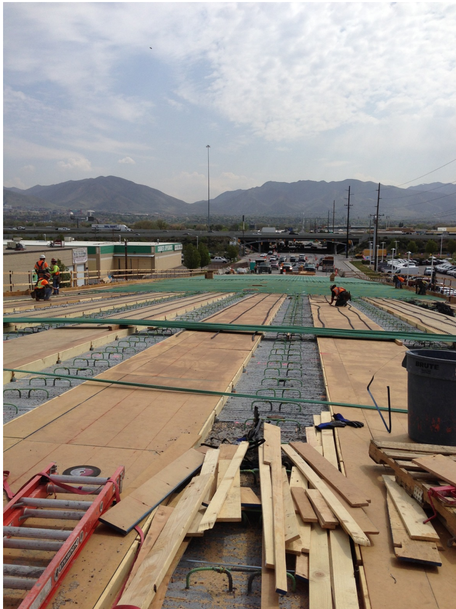
Forming the bridge deck
