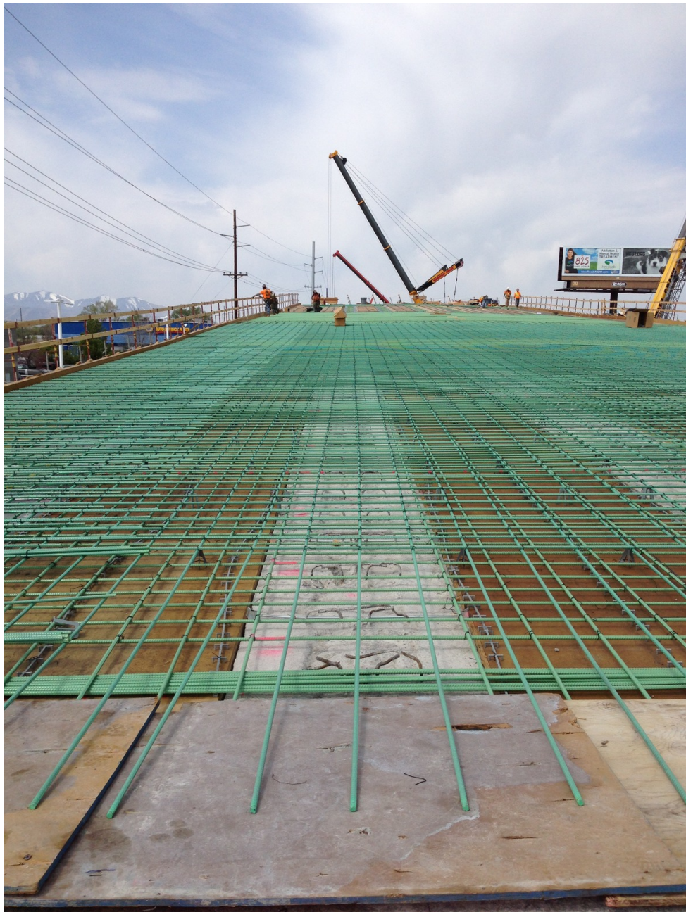
Rebar installation
