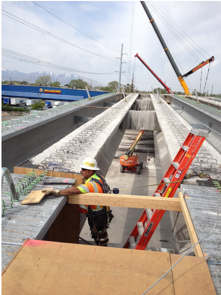
Forming the bridge deck
