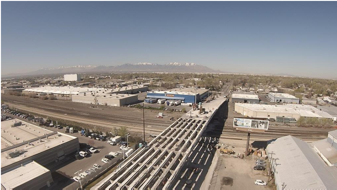
Aerial view of the project
