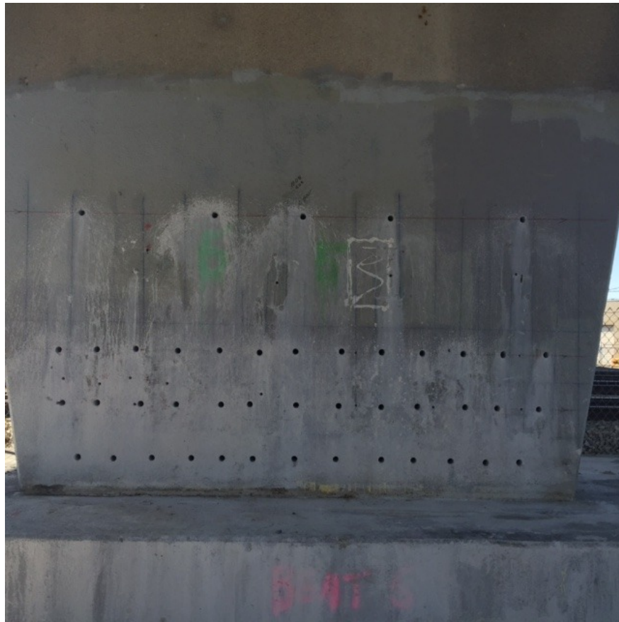
Holes drilled through the column
