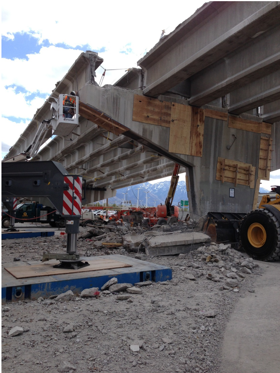
Repair work on the columns
