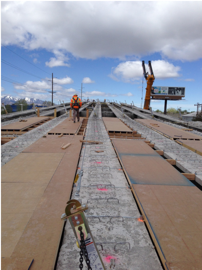
Forming the bridge deck
