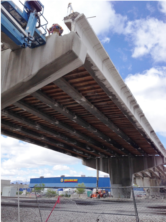
False bridge deck over the railroad tracks
